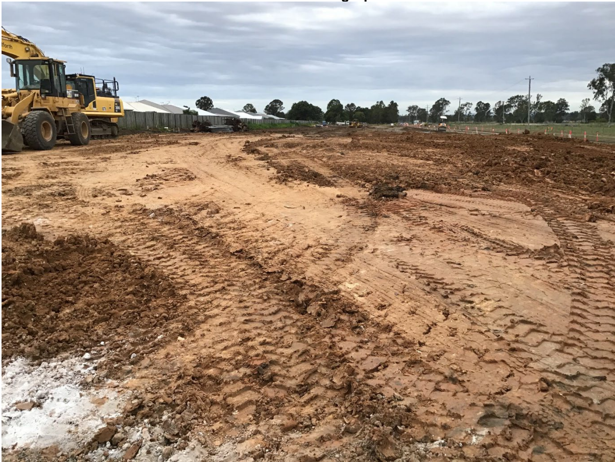
Picture 3: View of Filling Operations
