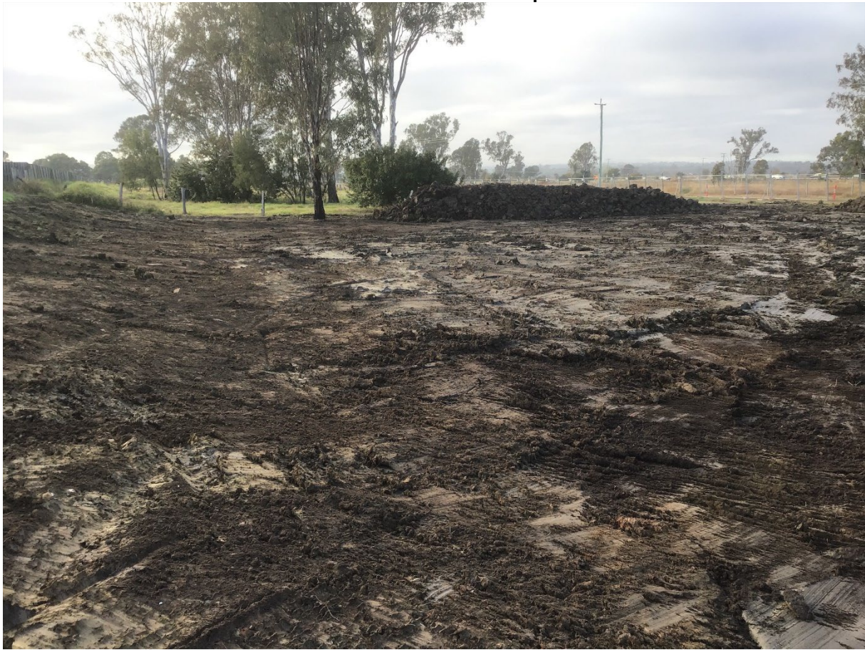
Picture 2: View of Earthworks Operations
